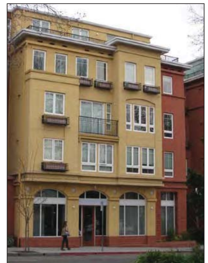
Image above shows office use on the ground floor with residential above
