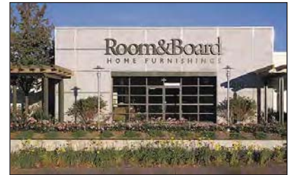
Above highlights a setback, articulated building that uses the setback space as plaza
