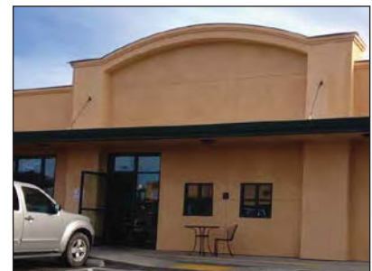
Unacceptable storefront entry
